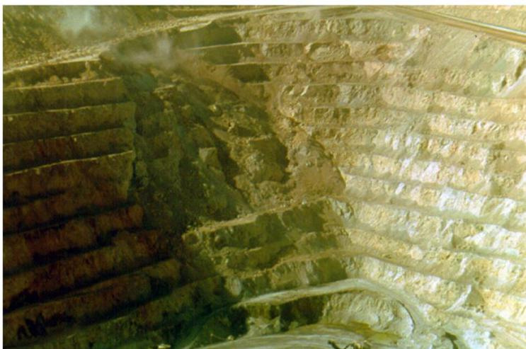
Figure 1: Mine slope failure (Hoek et al., 2000).
